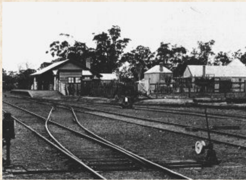
Typical Early GSR Station at Pingely (Photo ARHS Archives)
